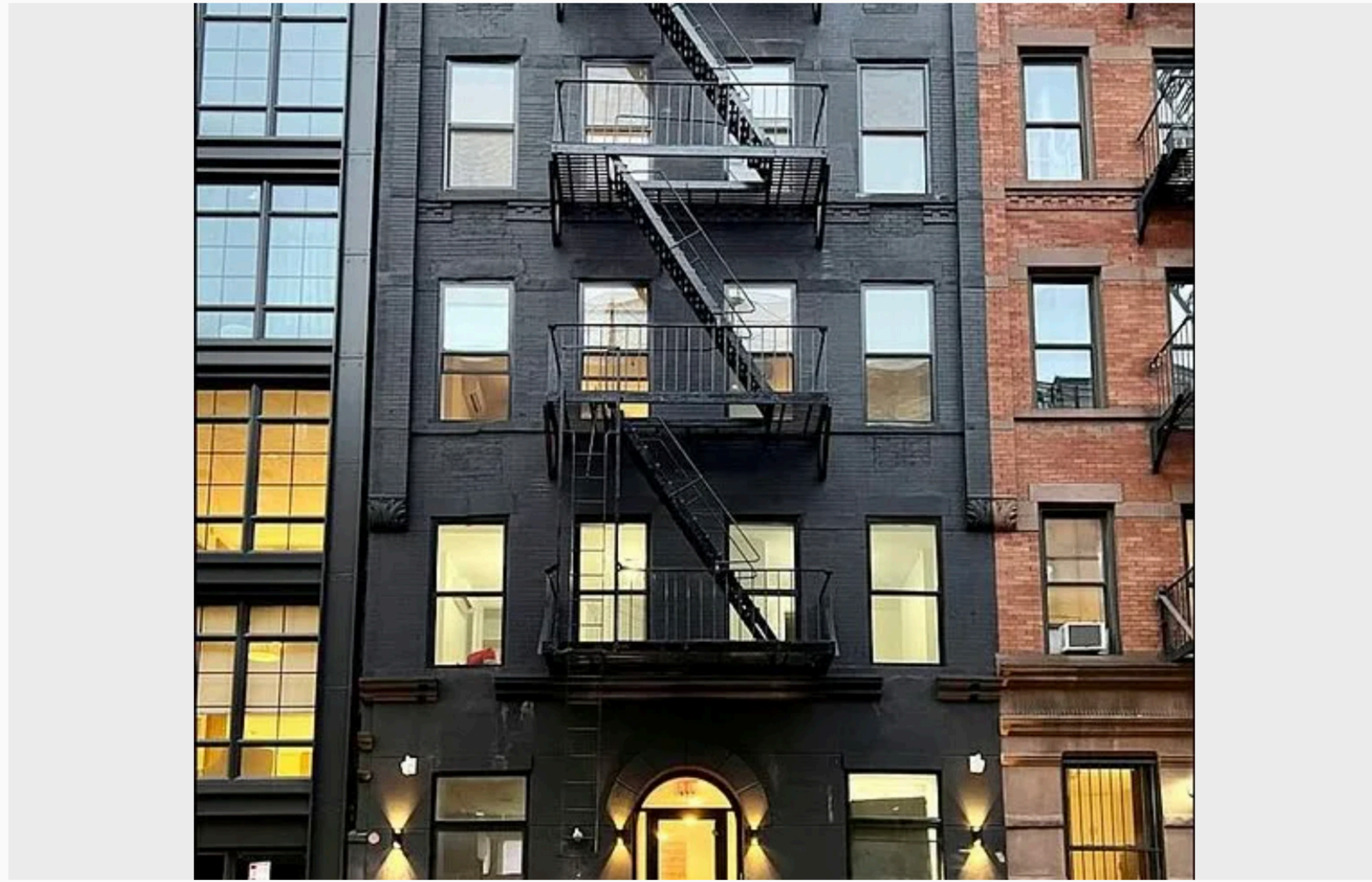
322 EAST 93RD STREET.
