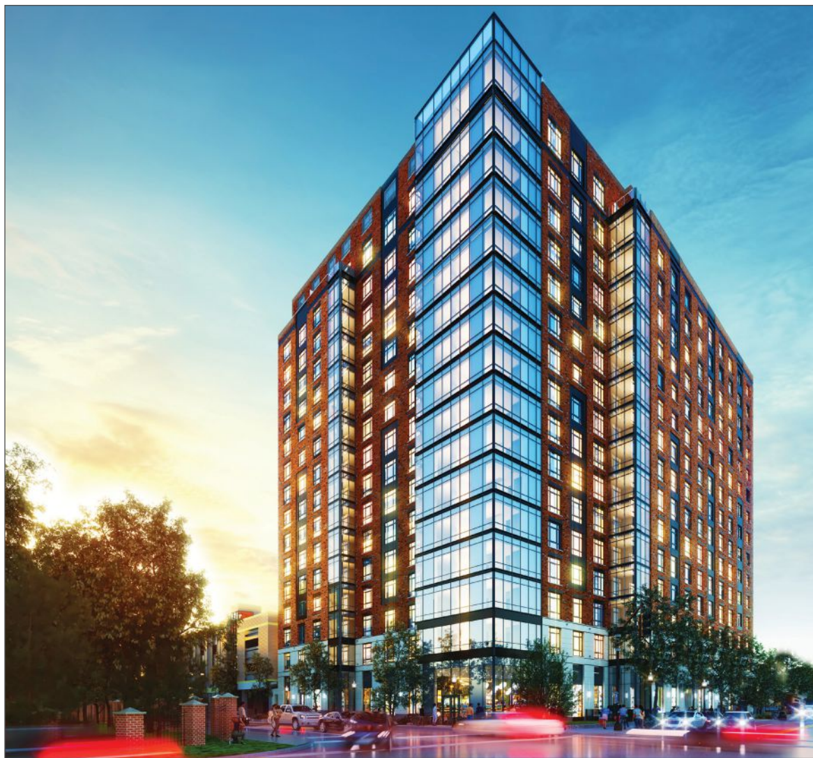
It took more than a decade to finish the 249 new apartments at 42 Broad St. in the Fleetwood neighborhood of Mt. Vernon, N.Y. The developer fought off two court challenges trying to stop the development.
