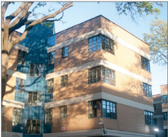
The new windows at the Williamsburg Houses in Brooklyn, N.Y., were custom-built to match the original windows at the historic landmark, originally completed in 1938.
